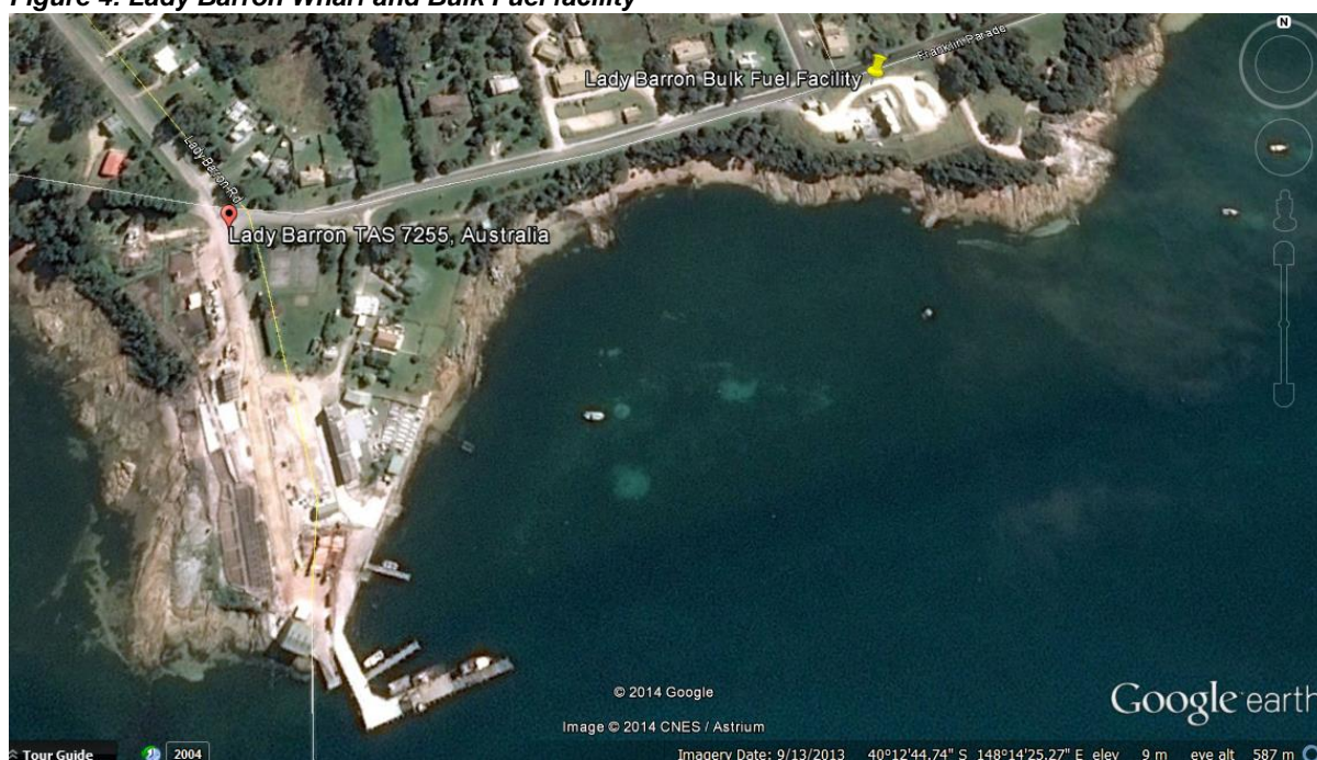
Figure 4: Lady Barron Wharf and Bulk Fuel facility
